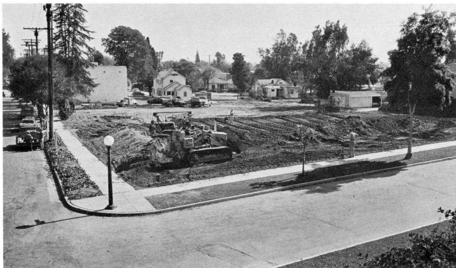
LEVEL BEGINNING—Tractors level ground for foundation as gymnasium construction begins.
